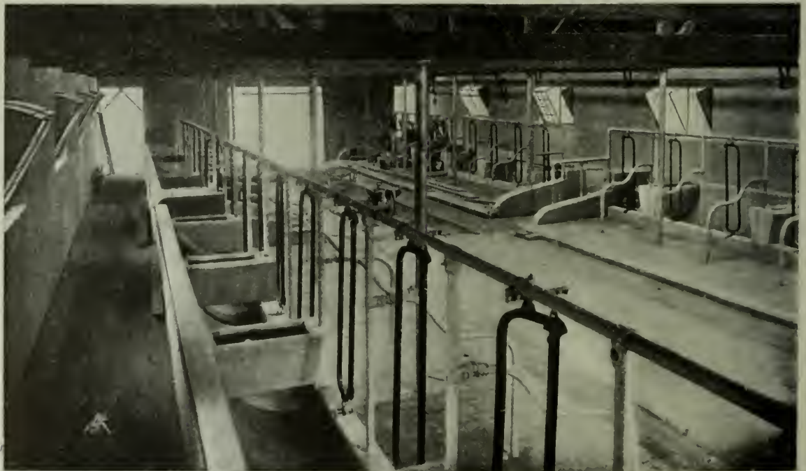
CONCRETE COW-BARN ON LORD ASTOR'S FARM, COOKHAM, BERKS : INTERIOR.
